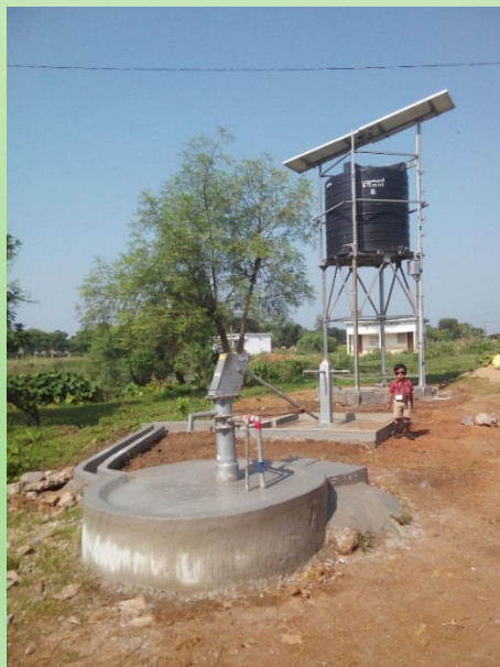
Solar pumps for drinking water
